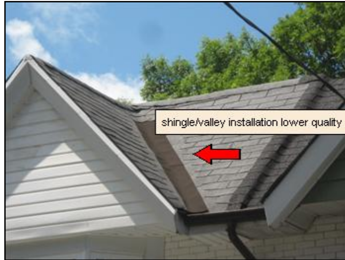
front sloped roof
