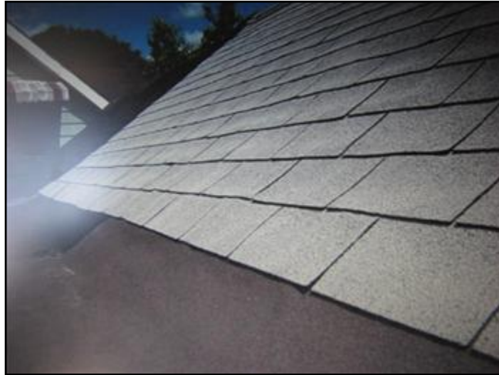
rear sloped roof
