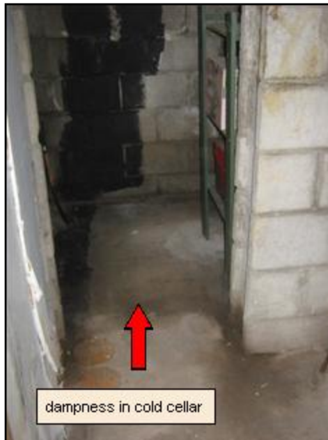
cold room under front stairs
