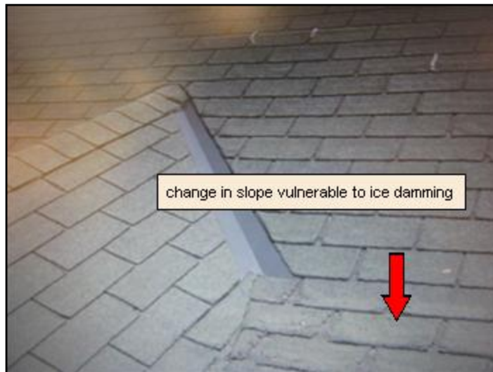
front sloped roof
