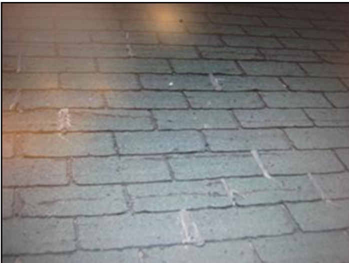
rear sloped roof
