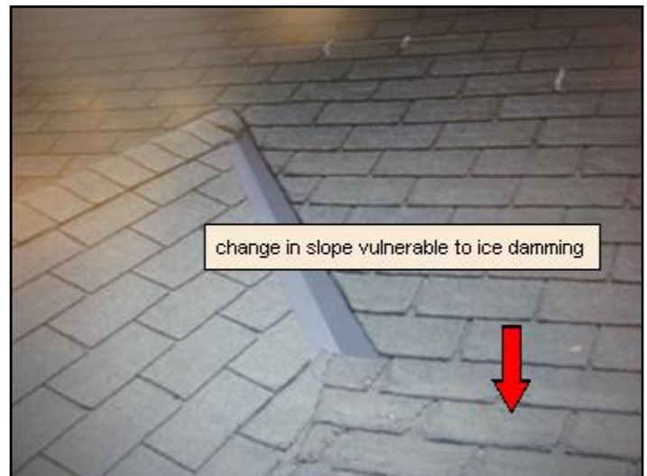
front sloped roof
