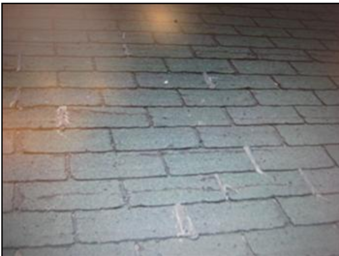
rear sloped roof
